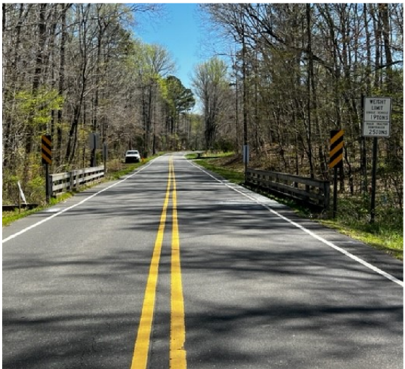
EAST APPROACH LOOKING WEST ALONG -L- ALIGNMENT
