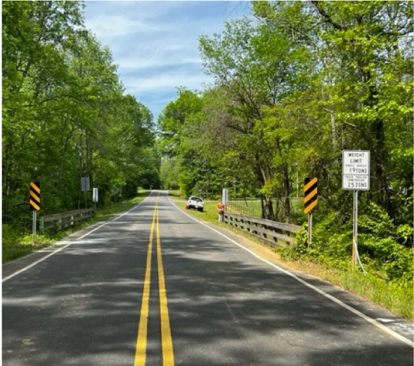
WEST APPROACH LOOKING EAST ALONG -L- ALIGNMENT
